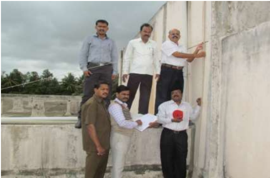
Water Tank Monitoring- Office Site
