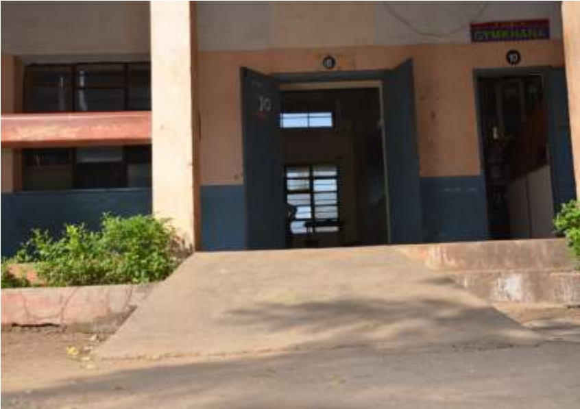
Ramps for Disabled students
