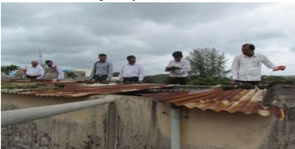
Water Tank Monitoring- Science building Site
