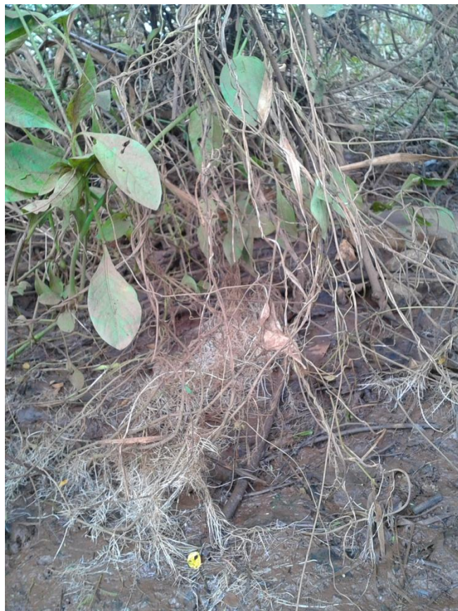
Photo Plate 8. Exposure of root system due to soil erosion by flood
