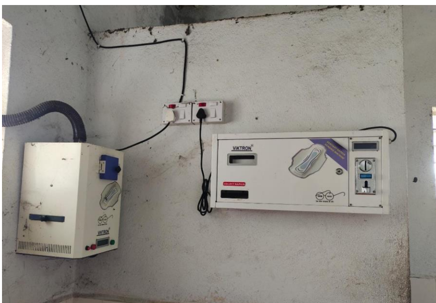
Sanitary Pad Vending Machine And incinerator
